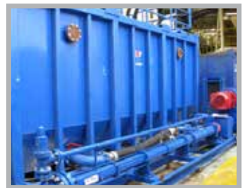
High Pressure hydro-cyclone feed for mud cleansing
